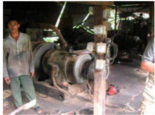
Picture 16: Existing REE Powerhouse
