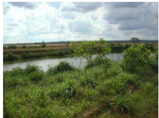
Picture 18: Effluent lagoon
