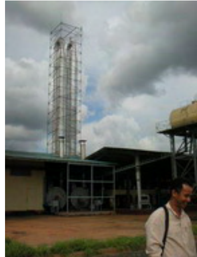
Picture 20: Starch powder drying column and boilers
