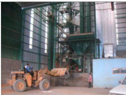
Picture 5: Grain drying silo structure
