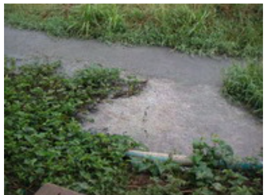
Picture 12: Open drainage channel from pens to lagoon
