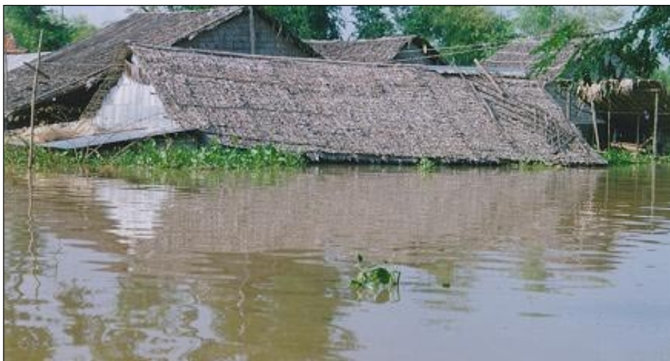
Photo 3: Roof top above flood water
