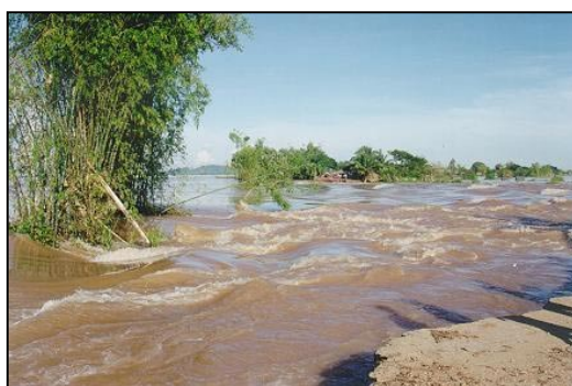
Photo 7: Road cut by flood waters
