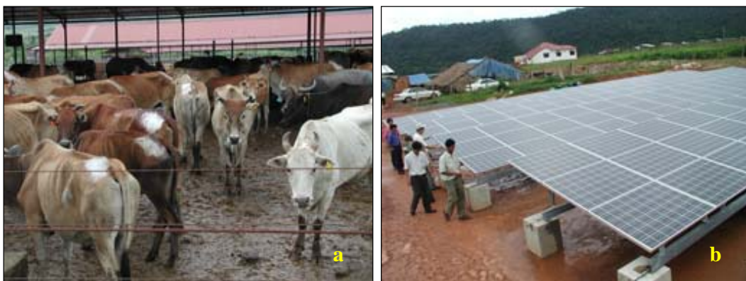
Picture 5: The 120kW Hybrid PV and Biogas Project near Sihanoukville: a) Cattle Manure Is Used to Produce Biogas, and b) Solar Energy Component
