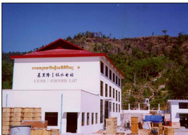
Picture 3: Kirirom 1 Hydroelectricity Power House
